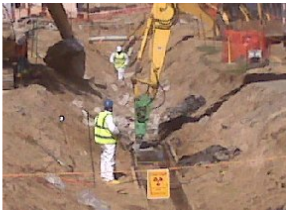
Figure 3 Cutting of Waste Transfer Pipes
