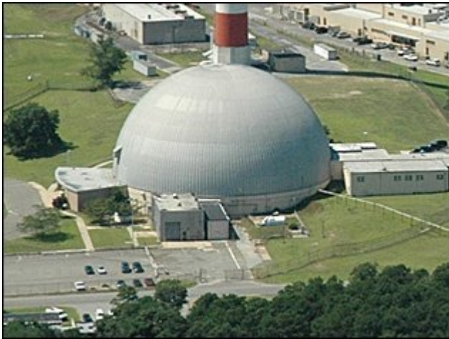
Figure 4 High Flux Beam Reactor Building and Stack
