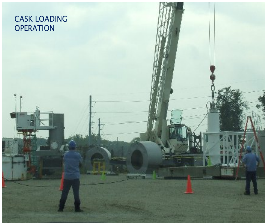
Fig. 3 Cask loading operation
