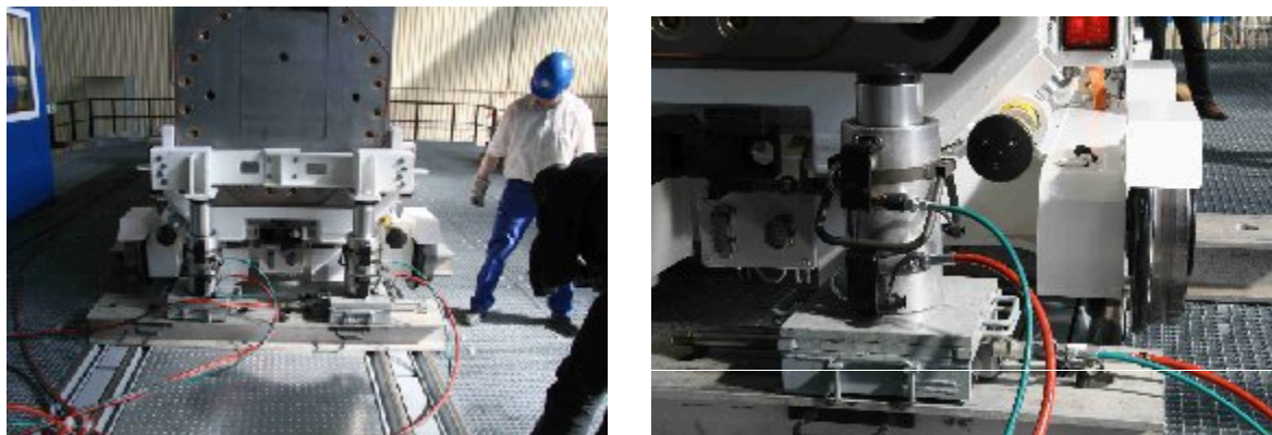
Fig. 12. Re-railing of the transport cart (left) and standard equipment (right)
