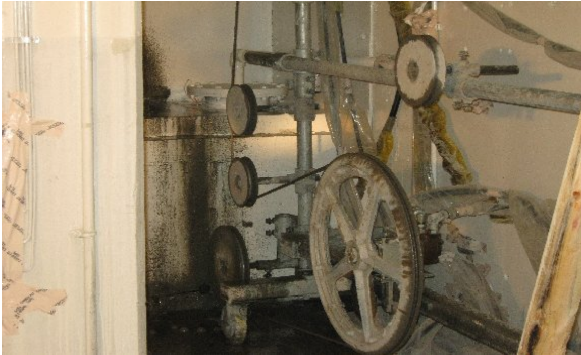
Figure 2. Wiresaw Cutting of Lower SERF
