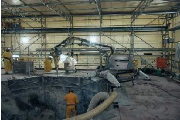
Fig. 9: Dismantling excavator in operation
