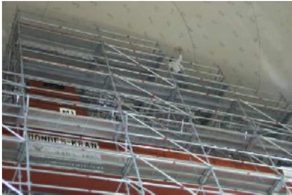
Fig. 19: Clearance measurements of the reactor dome
