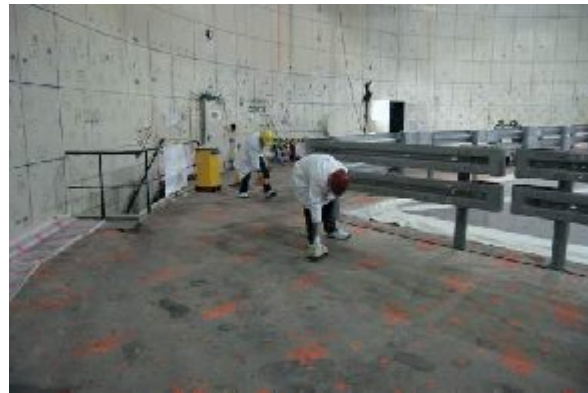
Fig. 20: Clearance measurements of floor and walls
