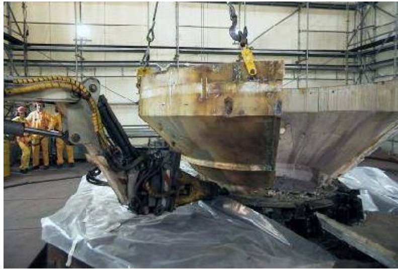
Fig. 12: Disassembling the thermal shield with dismantling excavator and rock chisel
