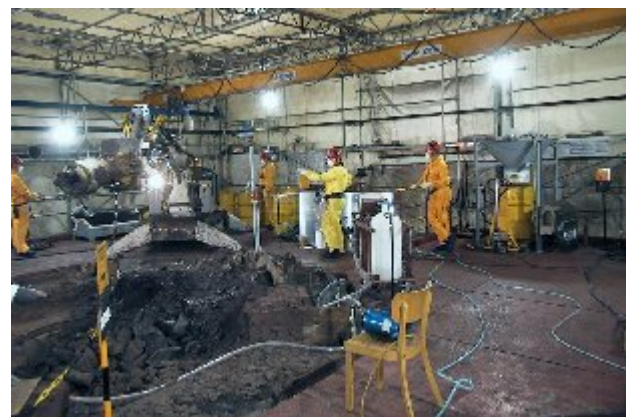
Fig. 14: Subsequent disassembly with the dismantling excavator
