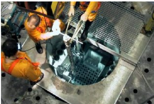
Fig. 2: Loosening a screw in the reactor tank
