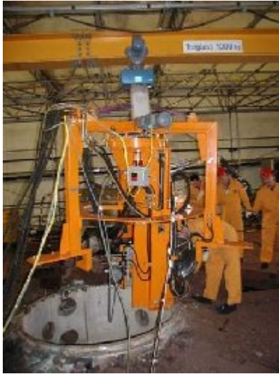
Fig. 11: Remote-controlled sawing device
