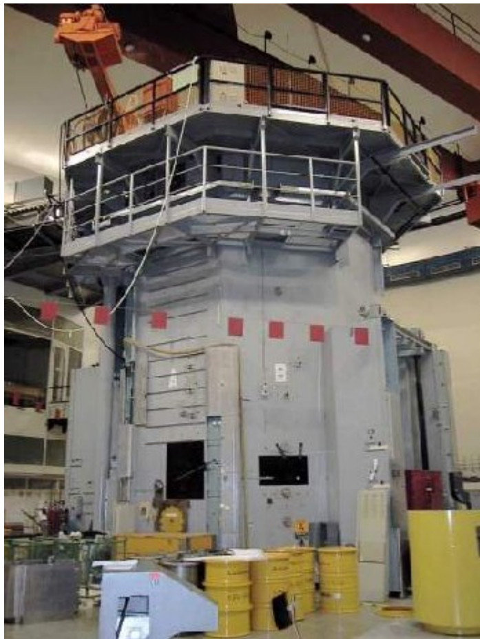
Fig. 8: Reactor block before disassembly
