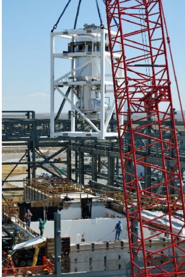
Fig. 2. The DMR vessel being lowered into place in the IWTU facility.
