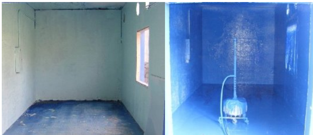
Figure 4. Hot cell mock-up interior before and after fixative spraying via whirling nozzle on remote platform.
