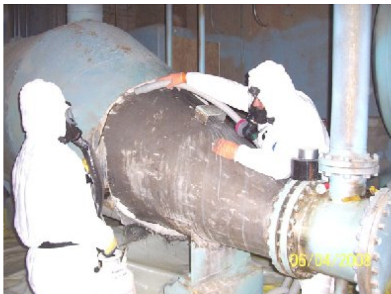
Fig. 1. In-cell asbestos removal activities in the Acid Recovery Cell.
