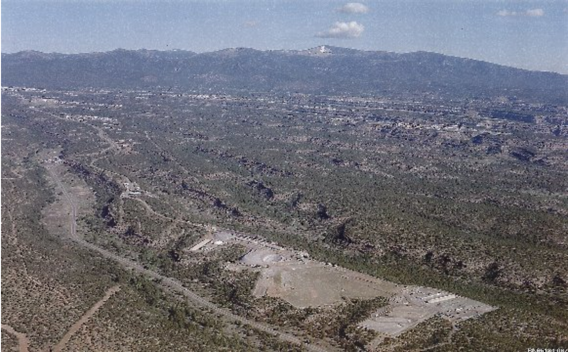
Figure 1. On-site waste Treatment, Storage and Disposal facility, TA-54, at LANL.
