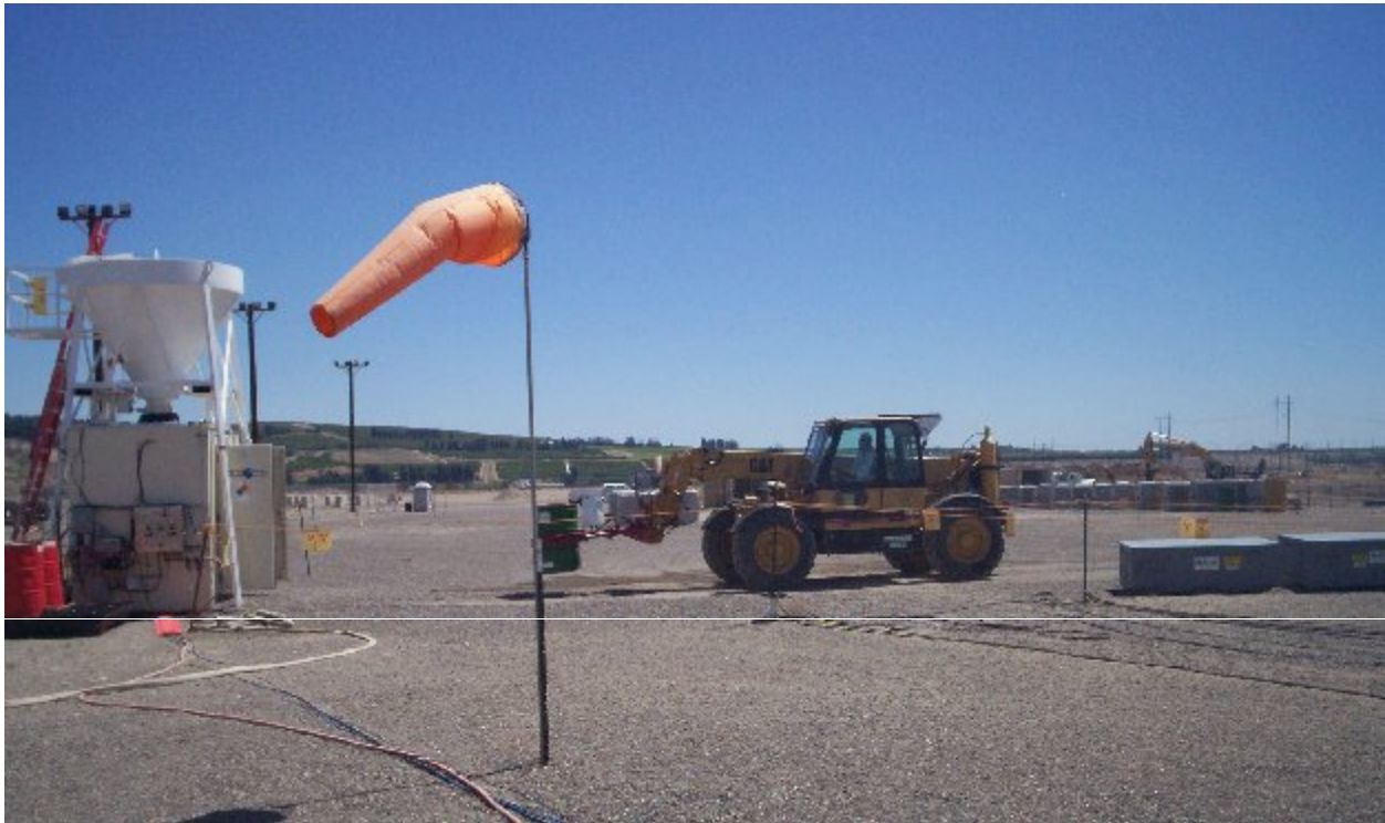
Fig. 3. Blast-shielded forklift transporting overpacked drum into drum punch facility.
