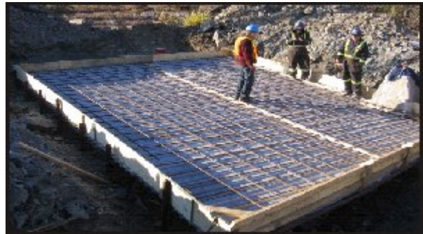
Fig. 4b. Capping of Mine Opening.
