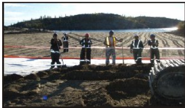
Fig. 4c. Engineered Cap at Silver Point.
