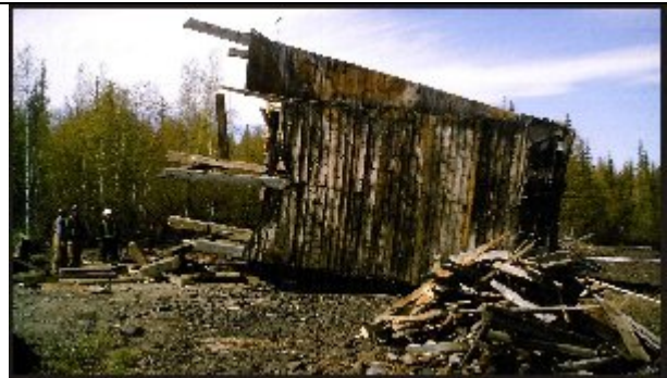
Fig. 3b. Cross Fault Lake Headframe Demolition.
