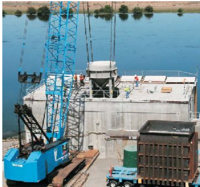
Figure 2. 96,000 pound box custom engineered for safe transport of contaminated filter tanks to the Environmental Restoration Disposal Facility.
