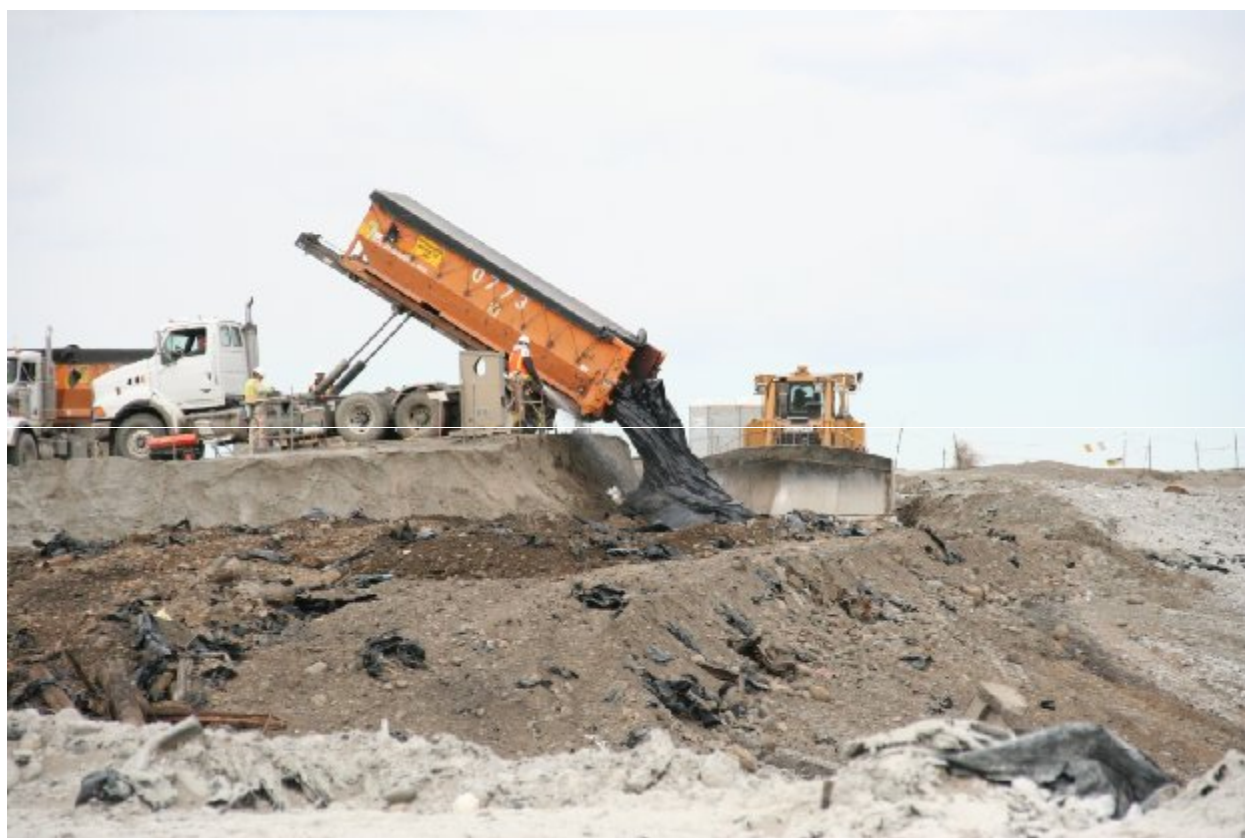
Figure 3. In the summer of 2009, disposal operations at ERDF averaged about 250 containers of waste per day. Upgrades underway will accommodate waste volumes more than twice the previous quantity.
