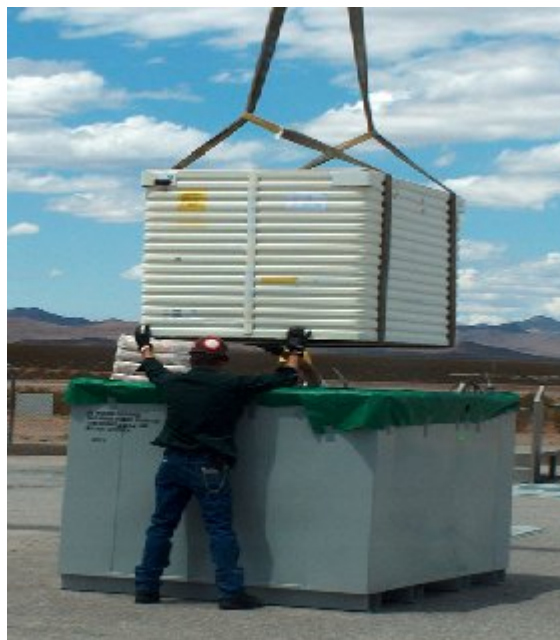
Fig. 4. Oversize box lowered into an UltraTech container before macroencapsulation.
