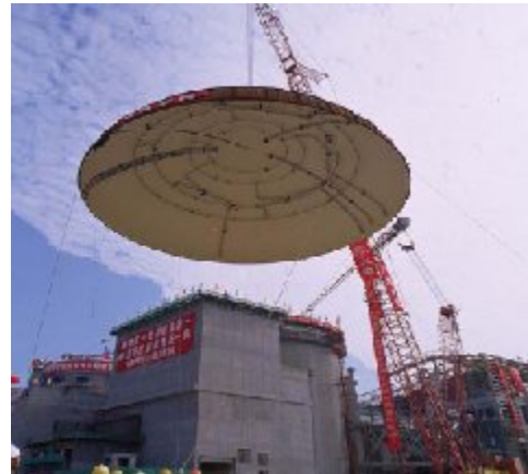
Figure 2: Lifting the dome module into place at Lingao-4 (from Reference [11])
