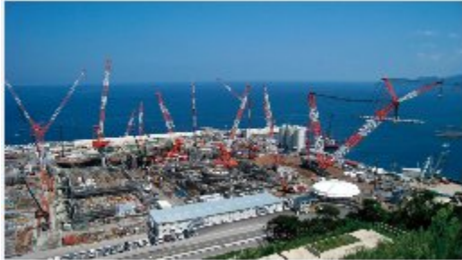
Figure 1: Shimane-3 Construction (Image courtesy: Hitachi)
