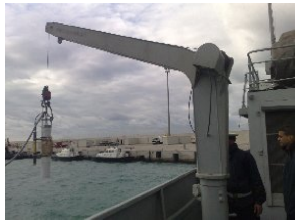
Fig. 8: Operation of the final installation of the fixed probe on buoy at the entrance of the Tanger MED port
