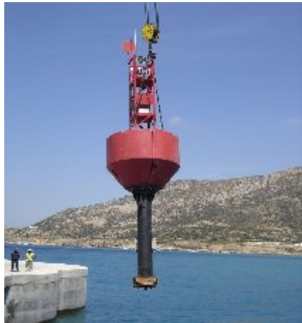
Fig. 8: Operation of the final installation of the fixed probe on buoy at the entrance of the Tanger MED port
