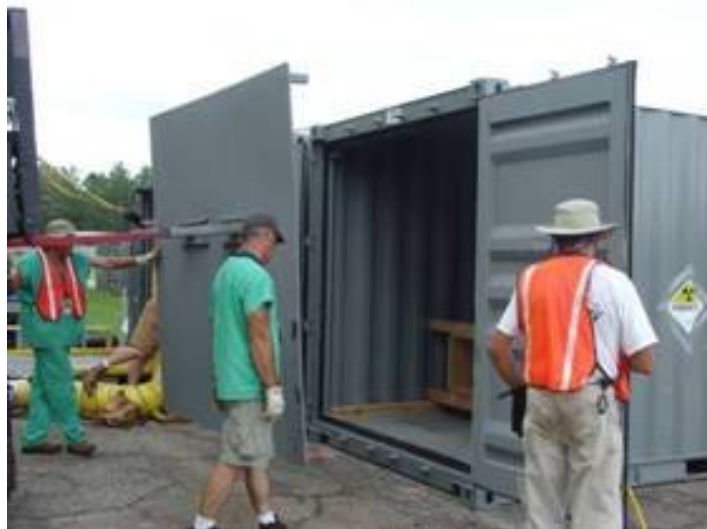
Figure 4 – Installation of bulkhead to seal door during Campaign 4.
