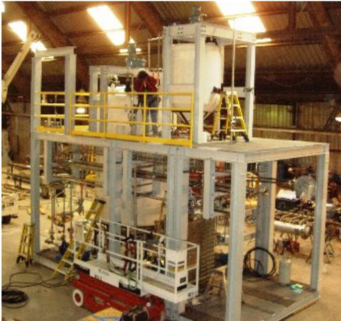
Fig. 3: Feed and shim vessel skid (P1) under construction
