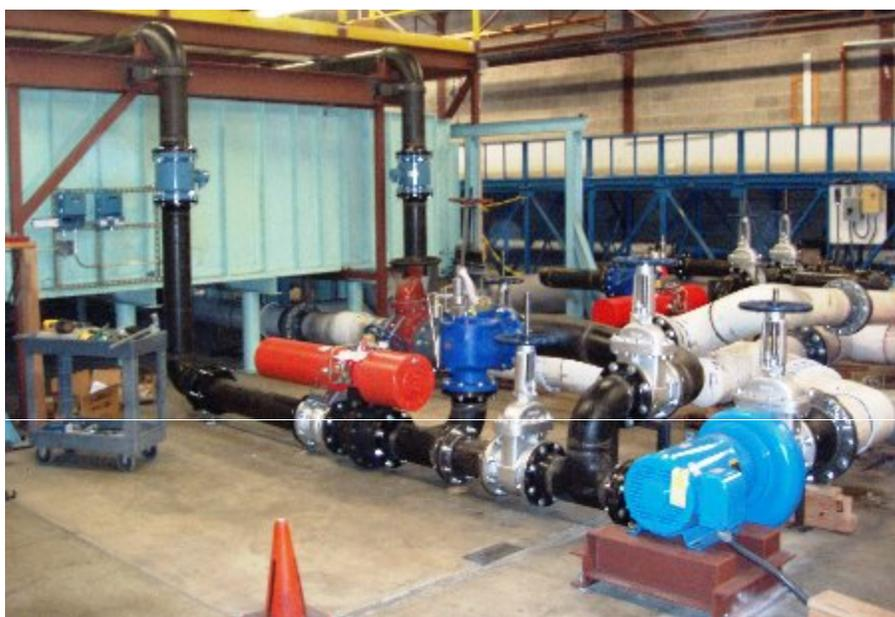
Fig. 9: Water feed system to the PJMs
