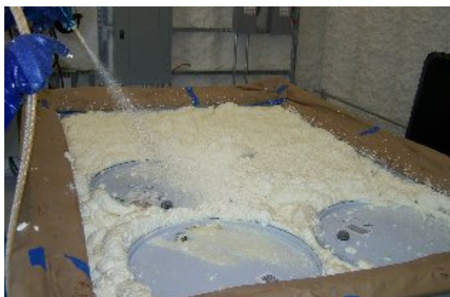
Fig. 3. Foam being added to fill void 2 .
