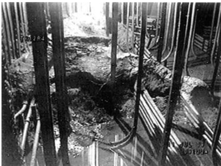
Fig. 4. Post-transfer video in Tank 12H reveals uneven topography and significant mounding. 11
