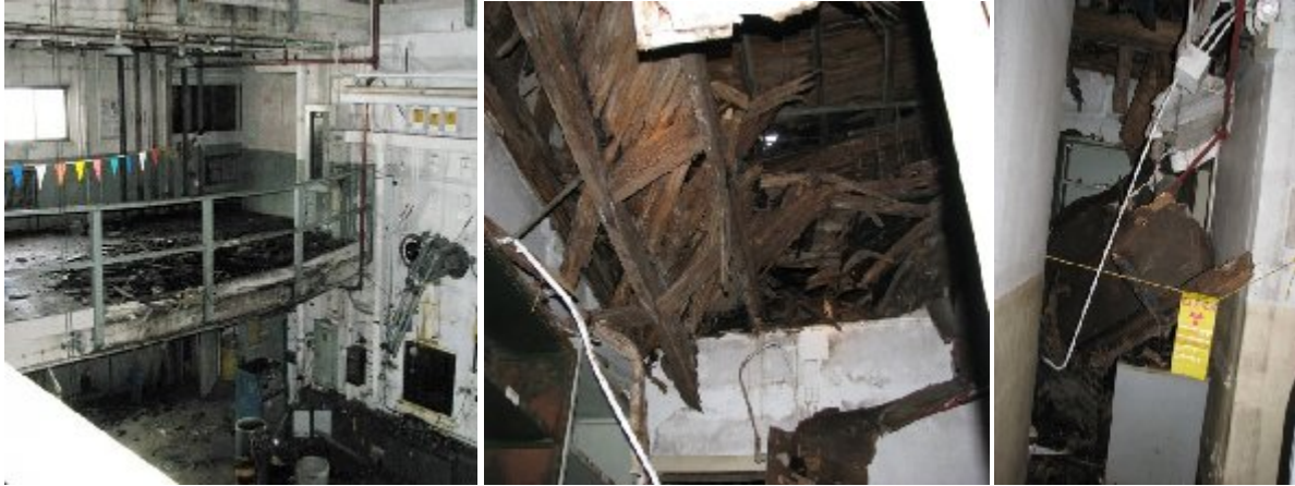
Fig. 4. Interior condition of 3026 at project initiation
