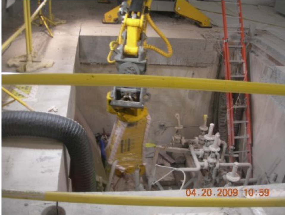
Fig. 4. Brokk 330 Demolition Robot in Operation at the TRA-613A Vault.
