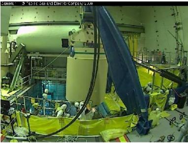
Figure 9 - Davit Crane Lowering HI-STAR HB into SFP
