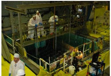
Figure 12 - Loading Fuel into an MPC
