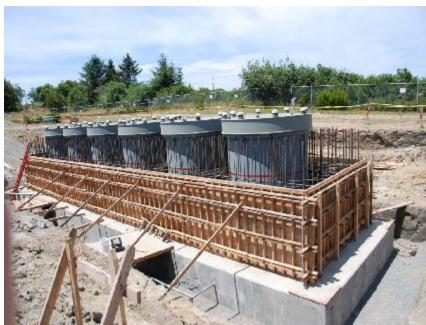
Figure 7 - Vault Liners in Place and Prep for Second Concrete Pour
