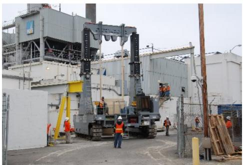
Figure 16 - Maneuvering the VCT out of the Radiological Controlled Area with a Loaded HI-STAR HB
