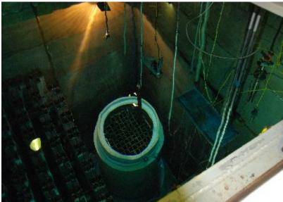
Figure 13 - Inserting a Fuel Assembly into a Submerged MPC
