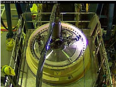
Figure 14 - Welding the Closure Lid onto the MPC Using the Automatic Welding Device
