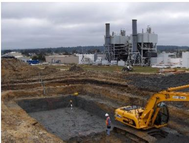
Figure 6 - Excavation for ISFSI Vault
