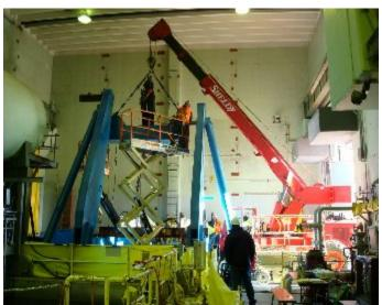
Figure 10 - Assembly of the Davit Crane in the Refueling Building
