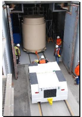
Figure 15 – Removing a Loaded HI-STAR HB from the Refueling Building Using the Airplane Tugger
