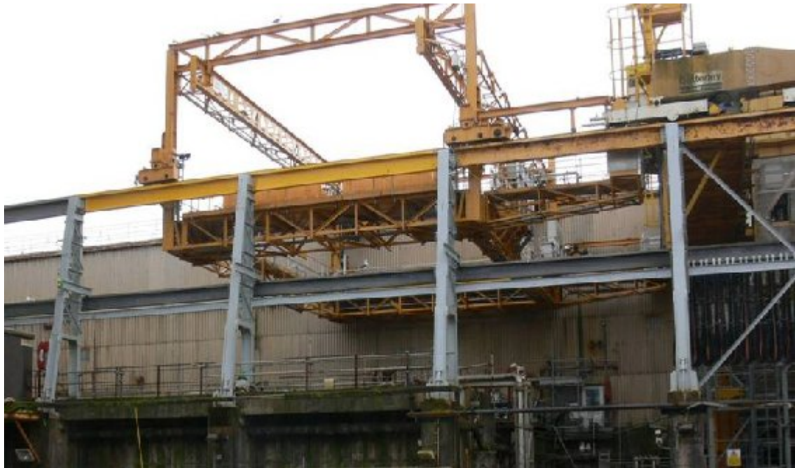
Fig. 5. The Gantry refurbishment system over the pond (the central yellow structure). To the right is the skip handler (also yellow)
