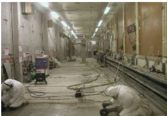
Fig. 3. Removal of Liners, Cut-off grinding
