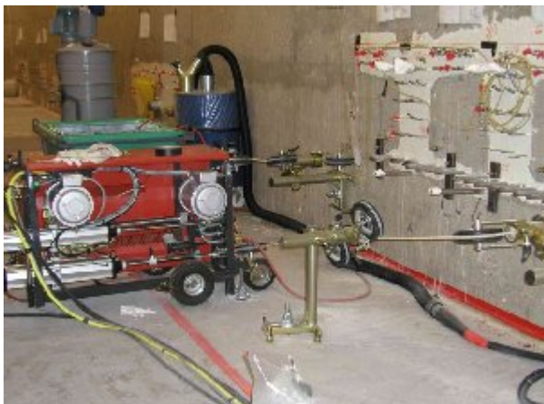
Fig. 1. Photographs of Removal of Feedthroughs
