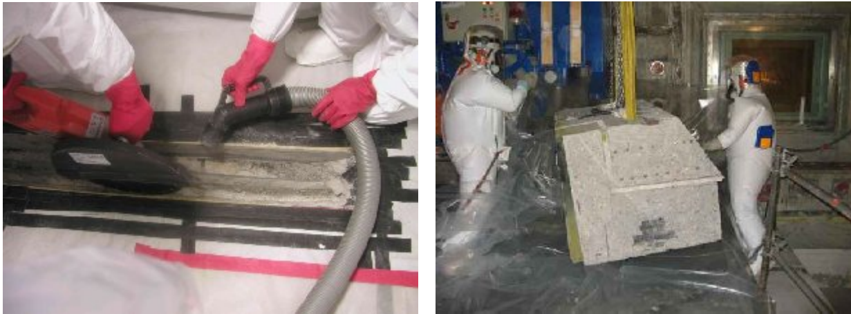
Fig. 2. Removal of Contaminated Building Joints
