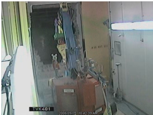
Figure 10: Remote wall breakthrough to the HWL
