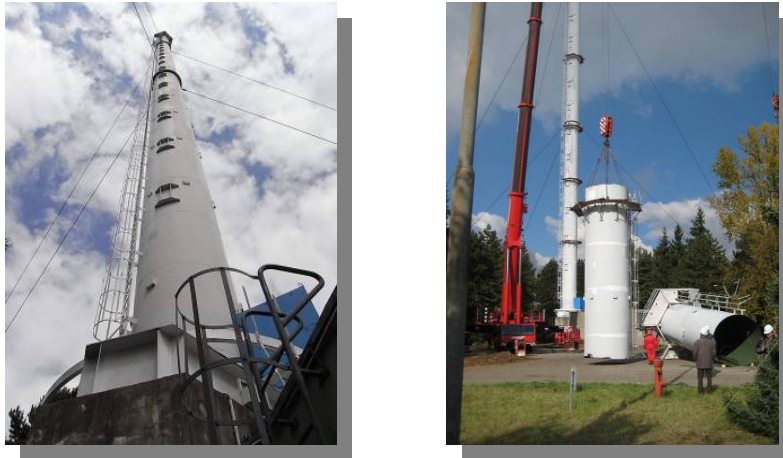
Figure 6: Shortening of the exhaust air stack down to + 18.5 m
