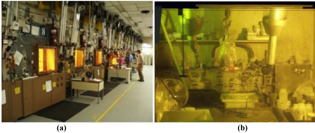
Figure 8: Photographs of (a) SRNL Shielded Cells Facility (b) RadBall Deployed in Hot Cell.
