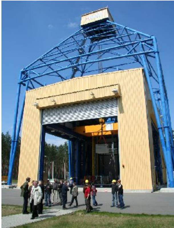
Fig. 2. The large 200 t BAM Drop Test Facility
