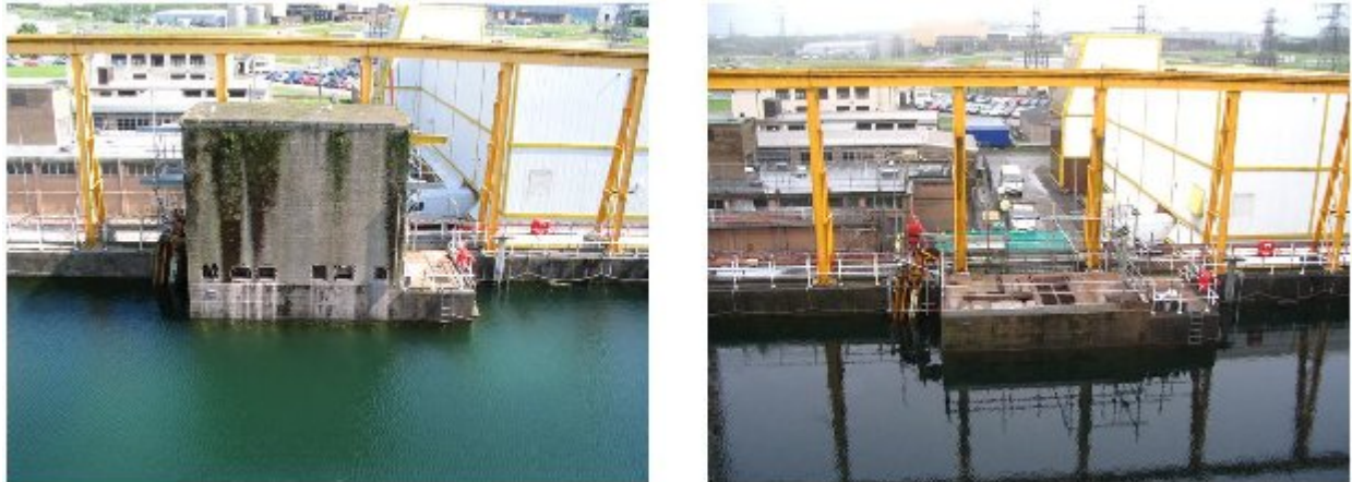
Fig. 3 East Winch House before and after demolition
