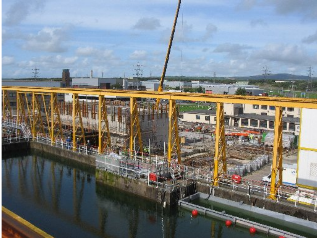
Fig.8. Construction of the Local Sludge Treatment Plant (Storage)
