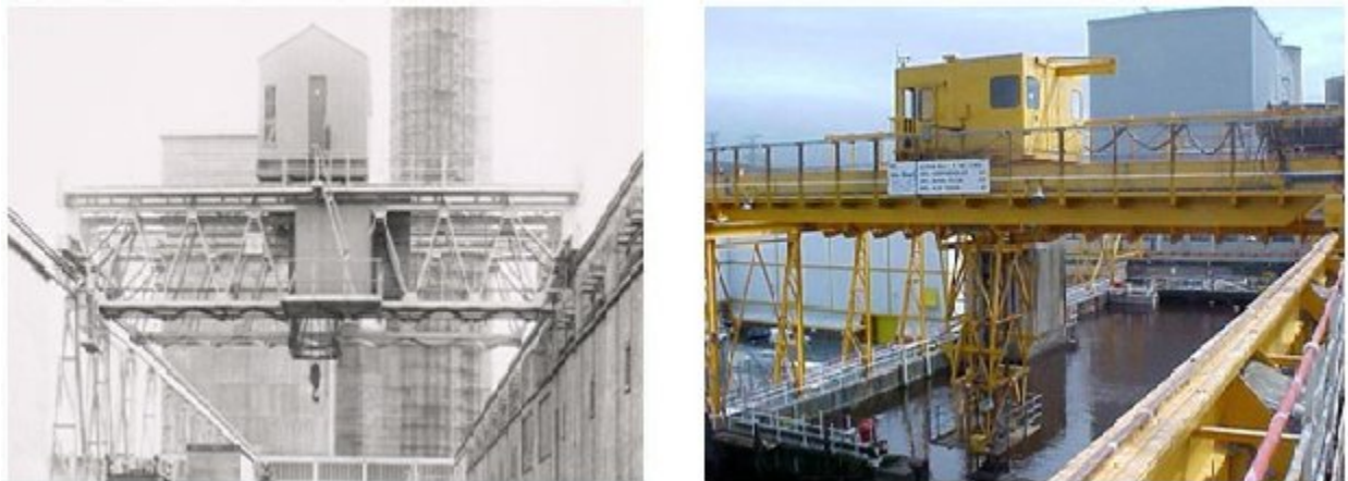
Fig. 2 Pile Fuel Storage Pond Skip Handler before and after replacement
