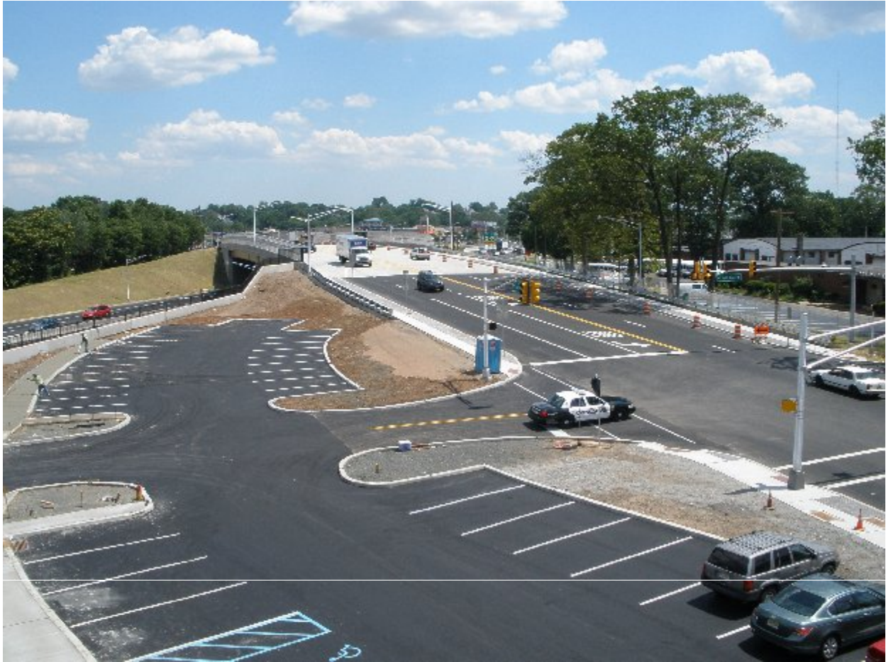
Figure 4. The restored parking lot at 99 Essex Street. The parking lot foreground was remediated and backfilled under FUSRAP. By agreement, NJDOT then restored the entire parking lot, including curbing, islands and striping, and the sidewalks shown here (photo courtesy of Joseph M. Sanzari, Inc.).
