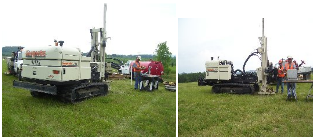
Figure 3. Geoprobe 8040 DPT rig used for monitoring well installation.
