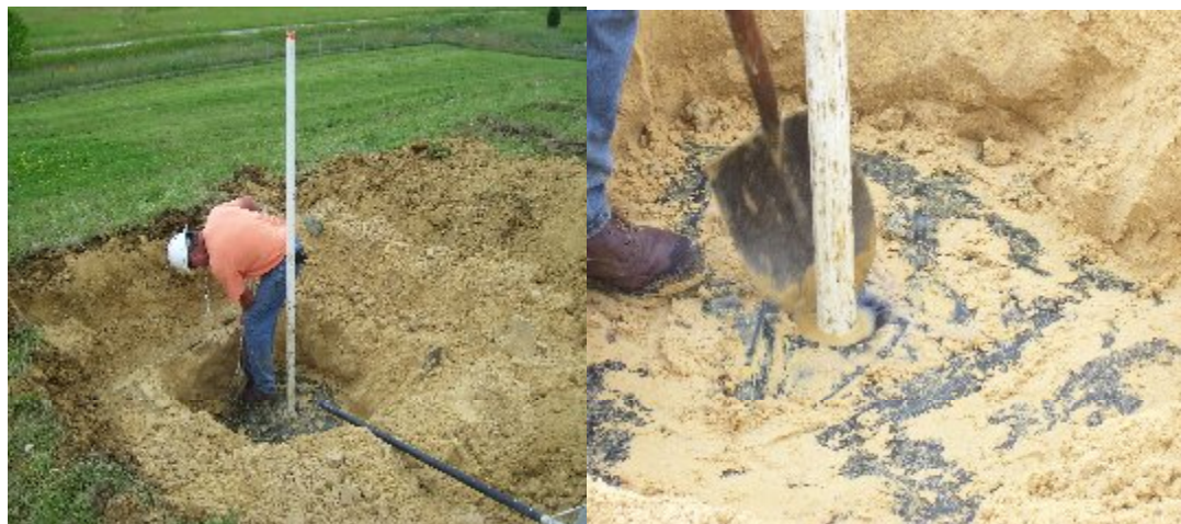
Fig. 4. Pipe boot being secured to landfill liner at monitoring well location.
