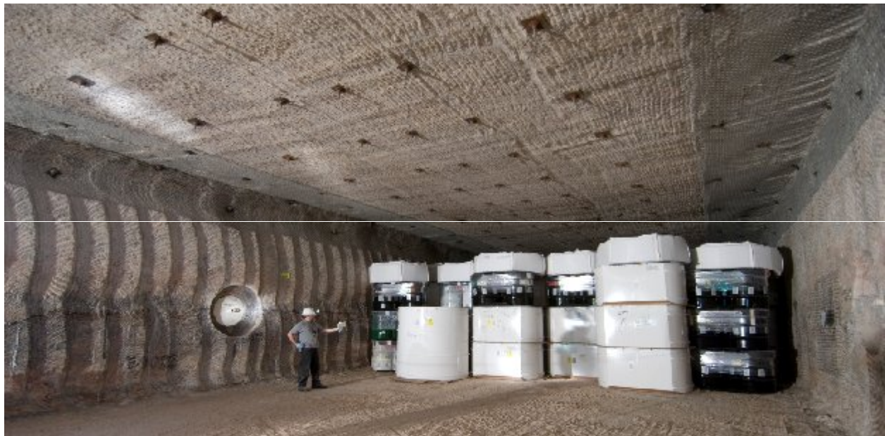
Fig. 4. Photograph of a disposal room in the WIPP repository. To the right of the man in the picture are different CH-TRUW containers with white super-sacks on top containing magnesium oxide (MgO). The MgO will stabilize the pH in the rooms after their closure. To the left of the man is the entrance of an emplacement hole for an RH-TRUW container.
