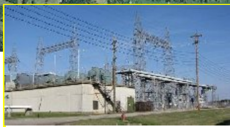
D&D of the X-533 Electrical Switchyard Complex
