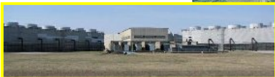
D&D of the X-633 Recirculating Cooling Tower Complex
