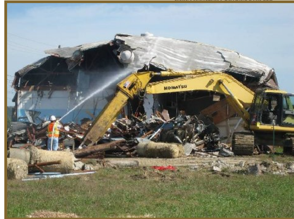
From 2006-2009, 17 inactive, surplus facilities were removed by LATA/Parallax
