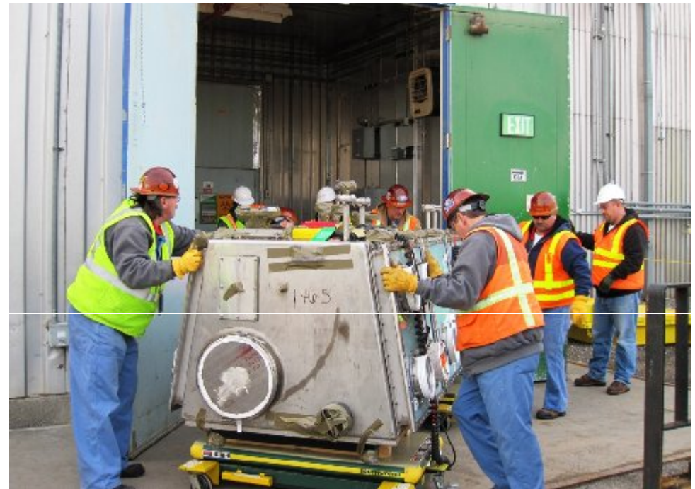
Glove box removal from the Plutonium Finishing Plant
