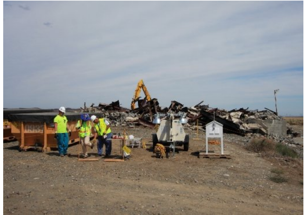
Demolition in the 200 North Area
