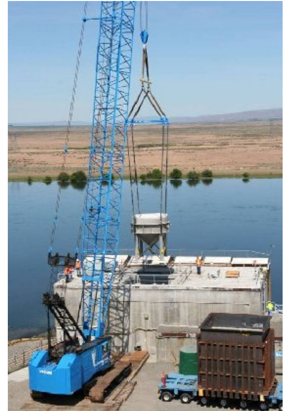
T-1 Tank removal
