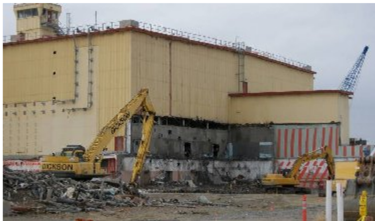
105N Control Room demolition
