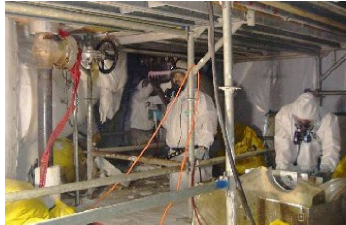
Asbestos abatement at N Reactor
