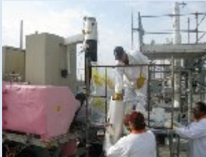
SY-P28 Exhauster removal (lead, asbestos, and radioactive material removal)
