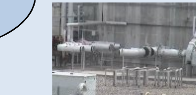
242-T HEPA filter removal
