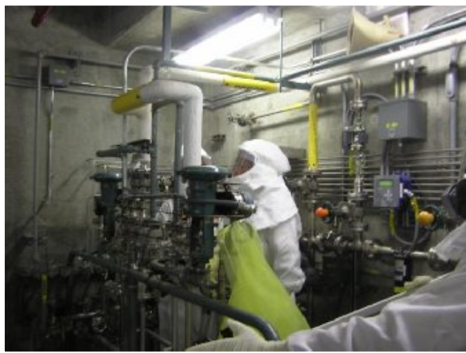
Left: 242-A Evaporator Valve Upgrade
