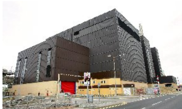
Residue Export Facility
