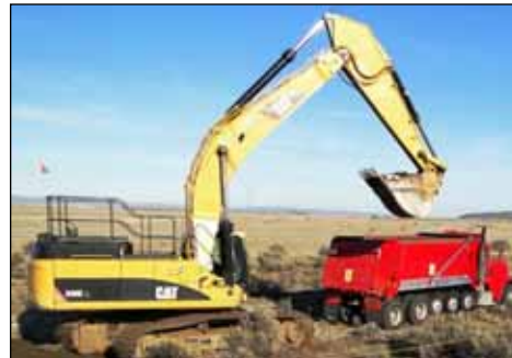
A super dump truck receives soil from a Hanford waste site.
