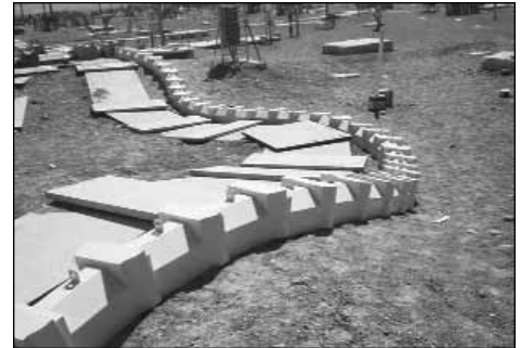
Shielded Hose-in-Hose Transfer Line in Hanford's 200 West Tank Farms
