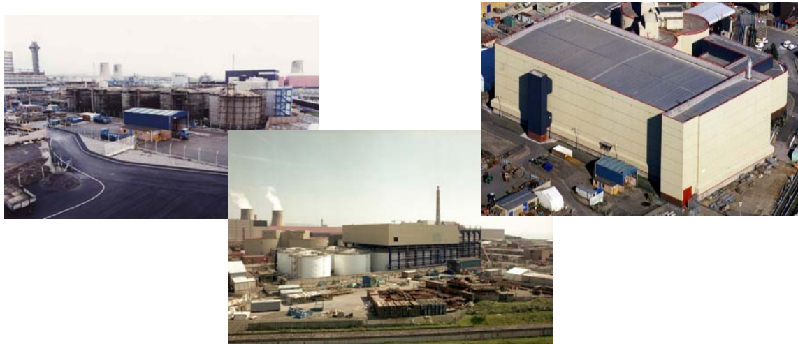
Figure 5 – Original uncovered tanks mid 80s → Overbuilding being slid into position late 90s → Completed overbuilding in 2000
