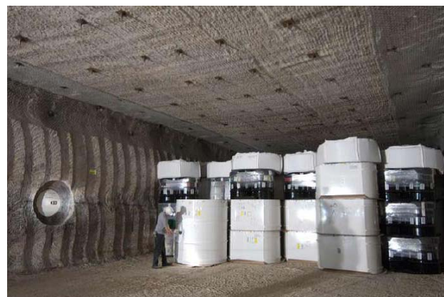
Fig. 5. Over 10,000 nuclear waste drums and standard waste boxes filling 1 of 56 rooms to be filled at WIPP over a 20-year period. Almost 25 rooms have been filled as of June 2008. Note the higher activity remote handled waste plunged into boreholes in the wall to the right and plugged with four-foot metal-wrapped cement.
