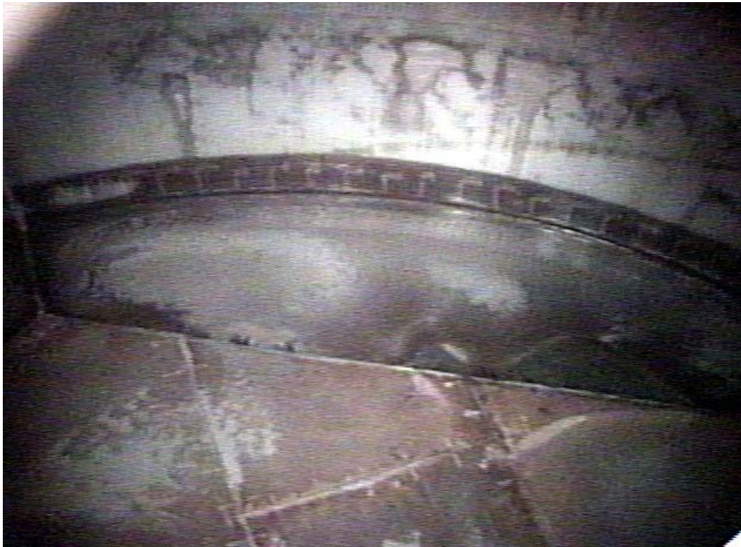
Fig. 3. TFF Tank WM-186 post-decontamination interior.
