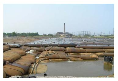
Fig. 4. The Consolidation Facility showing placement of filled geo-tubes.
