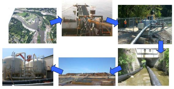
Fig. 2. Overview of sediment removal, transfer, de-watering, disposal, and water treatment process.
