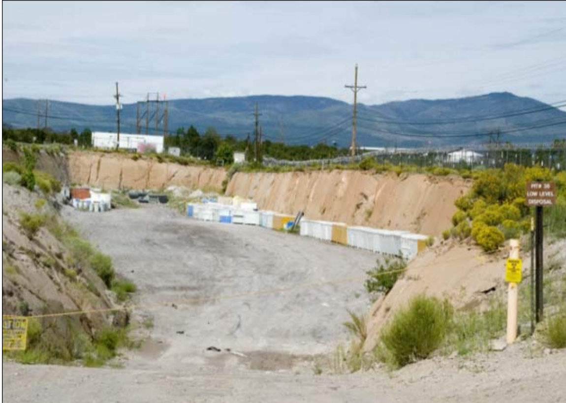
Figure 4. Active waste disposal pit at MDA G.
