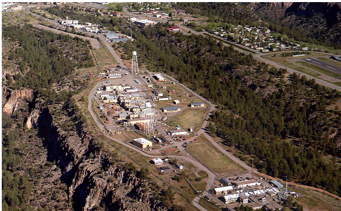
Figure 1. Aerial view of TA 21 circa 1995. MDA B is parallel to DP road at top left of photo.
