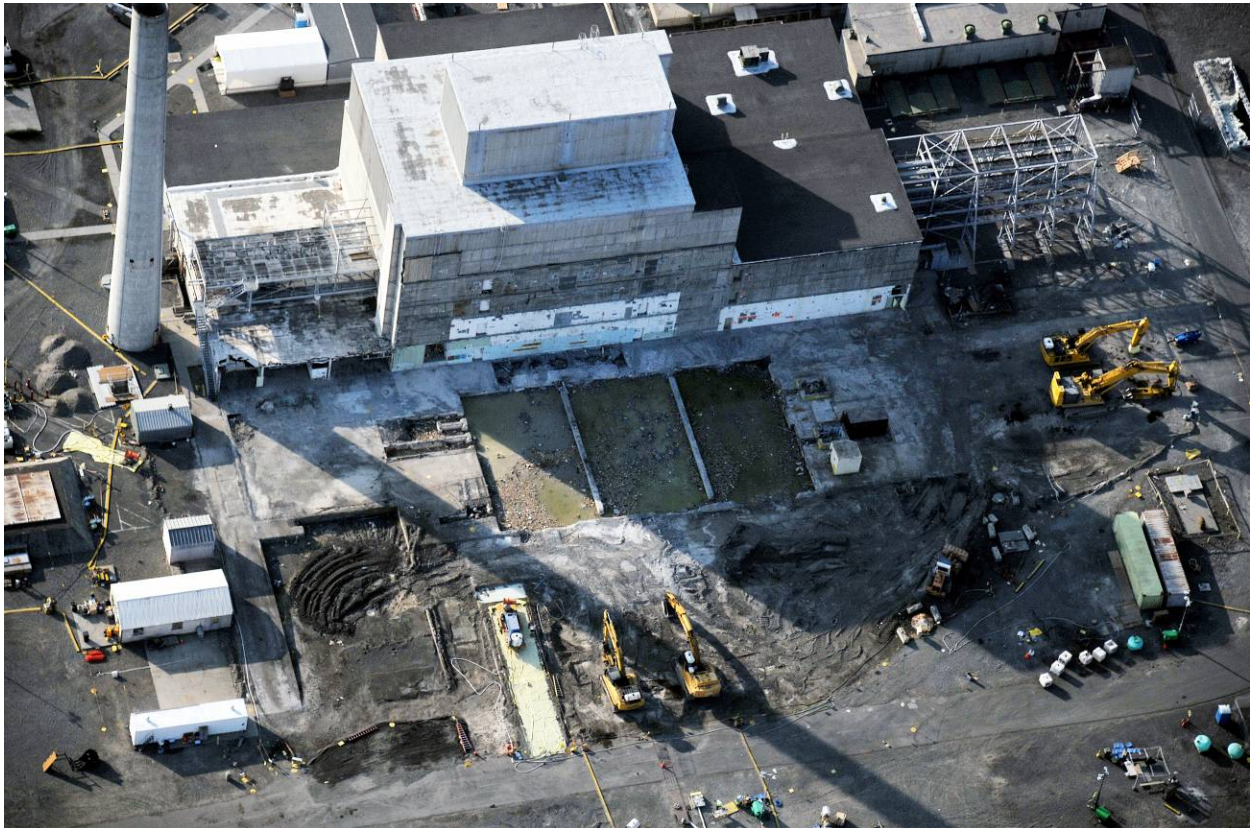
Fig. 4. The superstructure has been completely removed to slab-on-grade.
