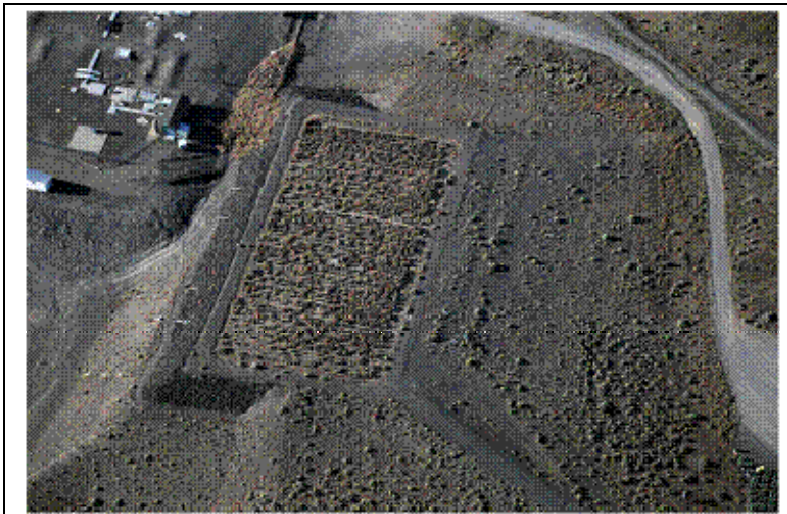
Figure 1. South Facing Aerial View of Prototype Hanford Barrier Showing Distribution of Plants on the Surface and Sideslopes. North is at the bottom end of the photo, south is at the top. Note the relatively sparse vegetation in the northwest (lower right) quadrant of the surface.
