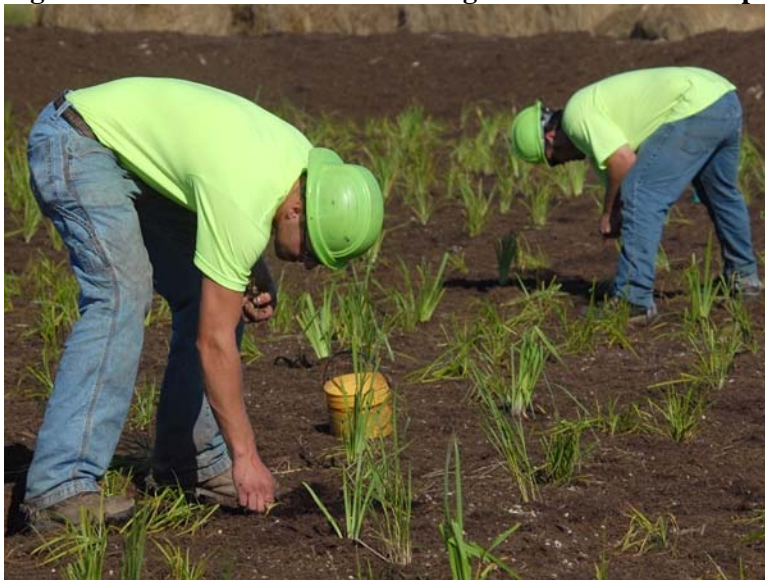
Fig. 1. The subsurface flow wetland gravel bed and mulch planting medium are being installed.
