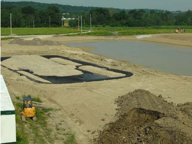
Fig. 3. The lined subsurface flow wetland sits adjacent to the larger surface flow wetland.
