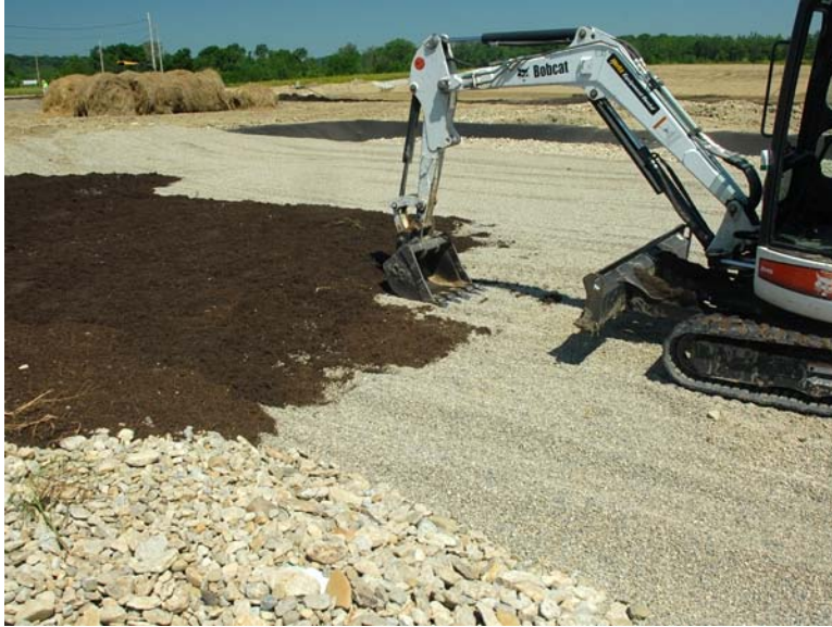
Fig. 1. The subsurface flow wetland gravel bed and mulch planting medium are being installed.
