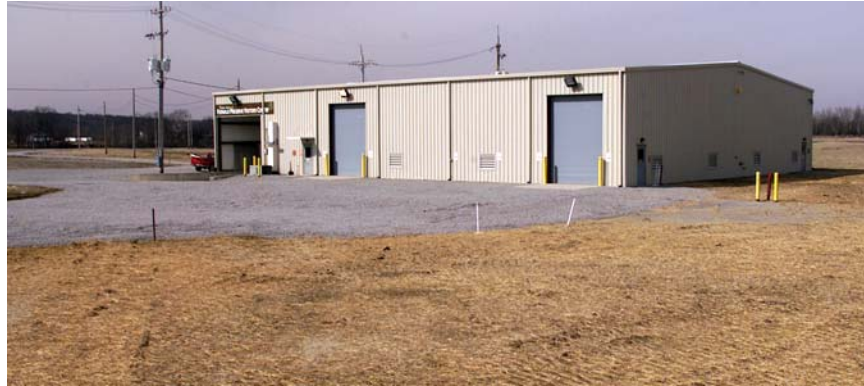
Fig. 2. Former Onsite Warehouse
