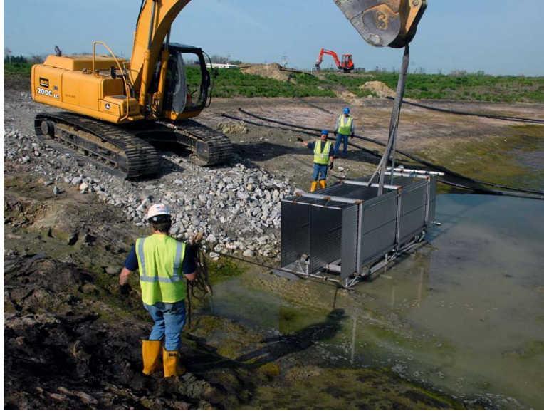
Fig. 4. Ground Source Heat Pump Installation
