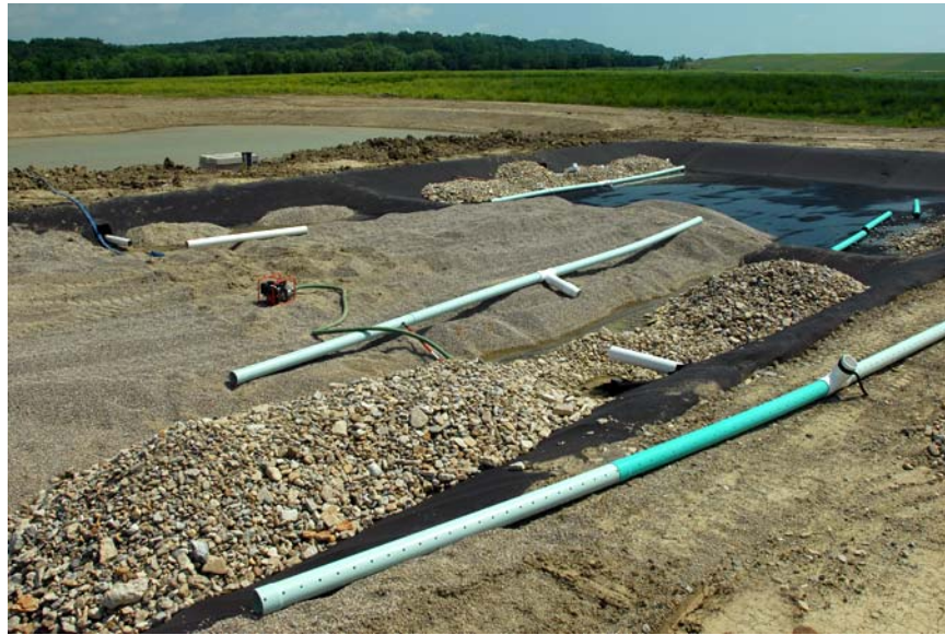
Fig. 3. Installation of Subsurface Wetland Piping and Substrate
