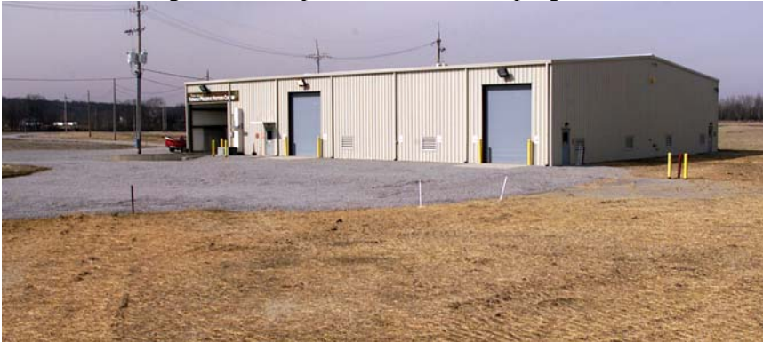
An existing warehouse was repurposed to become the Visitors Center
